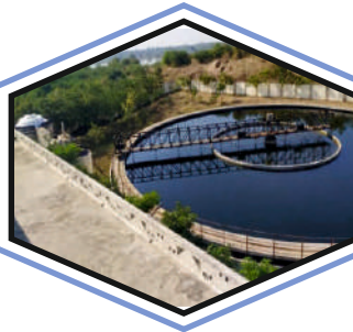
Sewage Treatment Plant Jetpur
